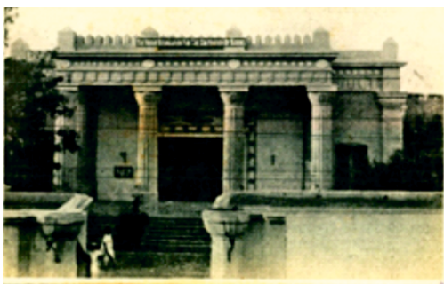
IACS building at Bowbazar Street, Calcutta
